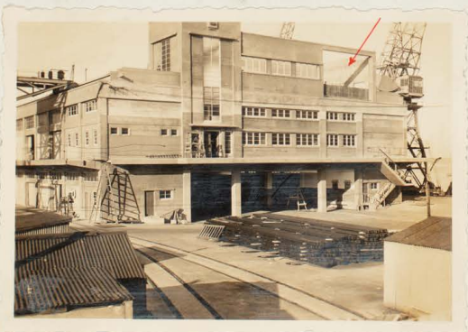
"View of Export Wharf Showing opening for Bridge at roof level."
