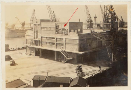
"View of Export Wharf from Cool Store." The Bridge portal enters the large opening on the face of the Building at Roof level.
